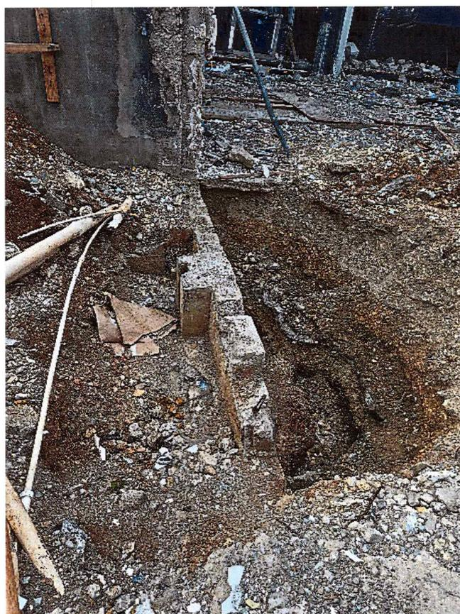
**IMAGEN 28: ZAPATA DE LA COLUMNA ELIMINADA EN ESCENARIO.**
